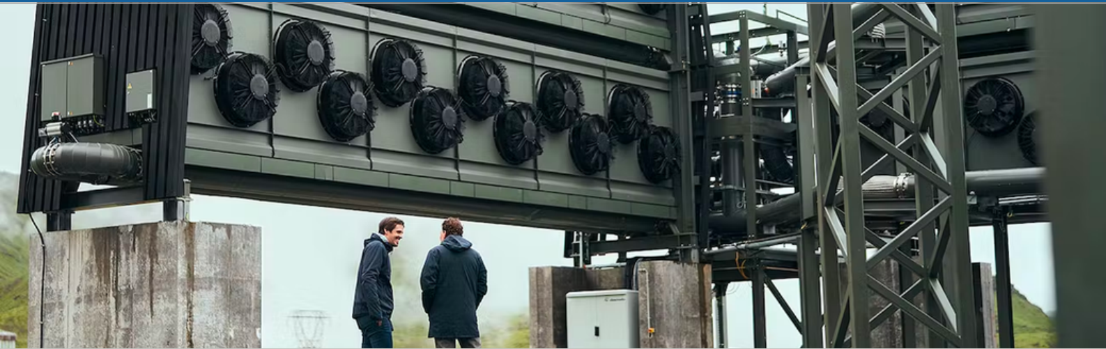
Orca, the world's largest direct air capture and storage plant that permanently removes CO 2 from the air, in Iceland. Credit: Climeworks
