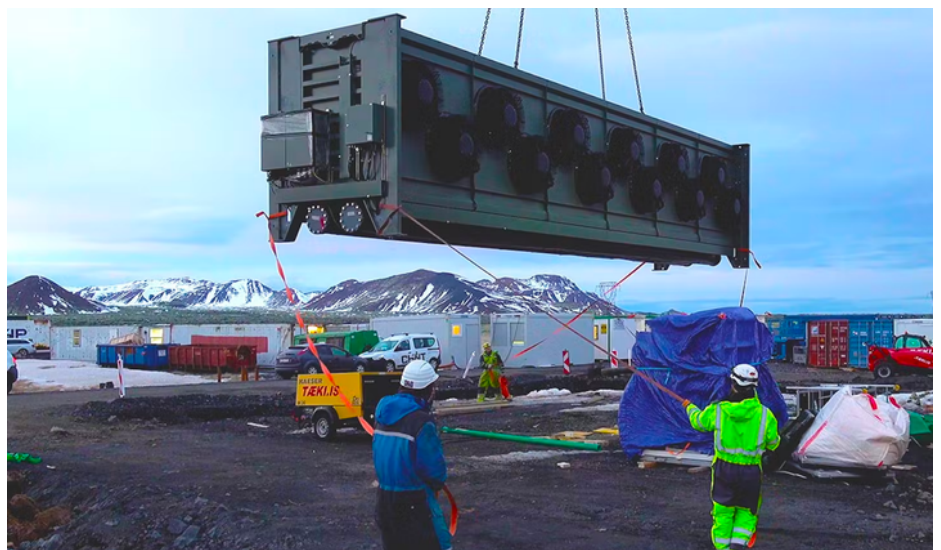
The first collector being lifted by a crane. Credit: Climeworks.
